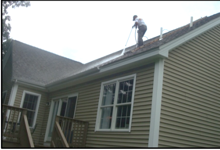
Roof washing on MacPherson's house.
