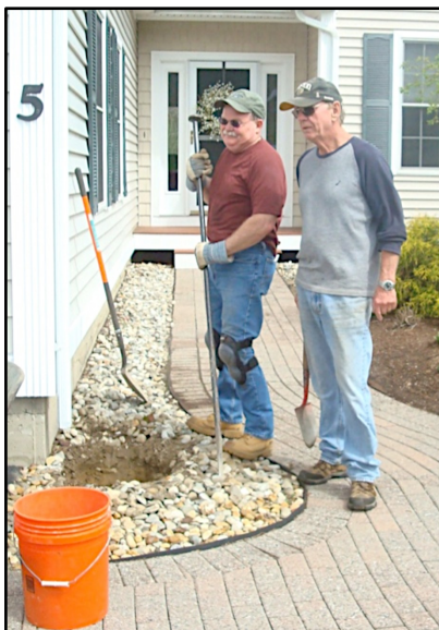
Paul Currier and Jack Bilodeau repair a storm drain.
